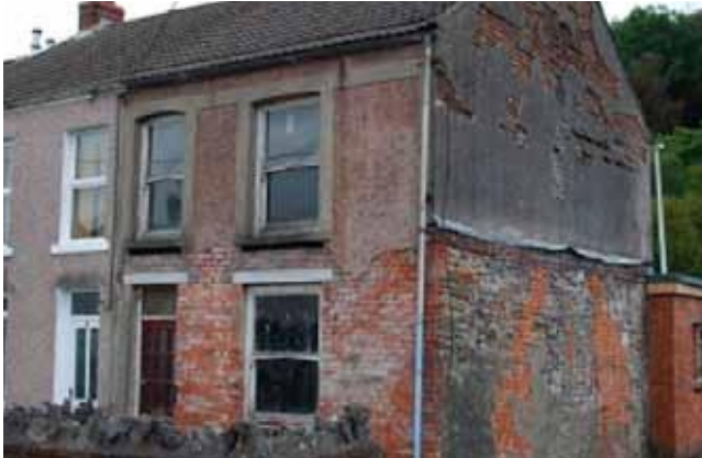
Before and after, photo: Julian Preece, Powys County Council
